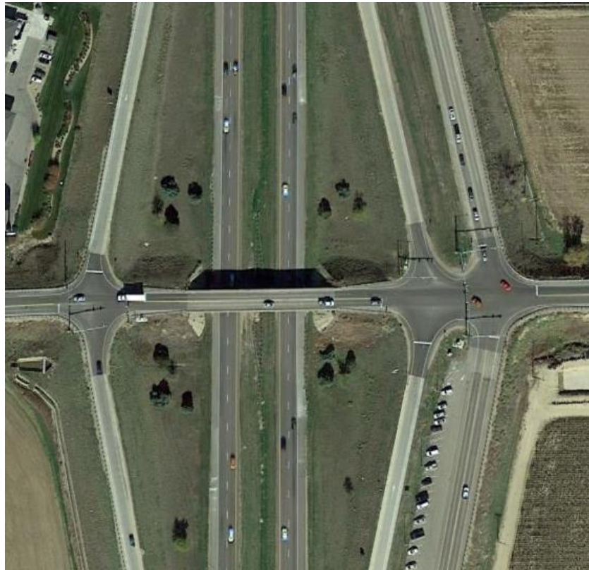
Figure 2. Current Condition of SH 60 Interchange
