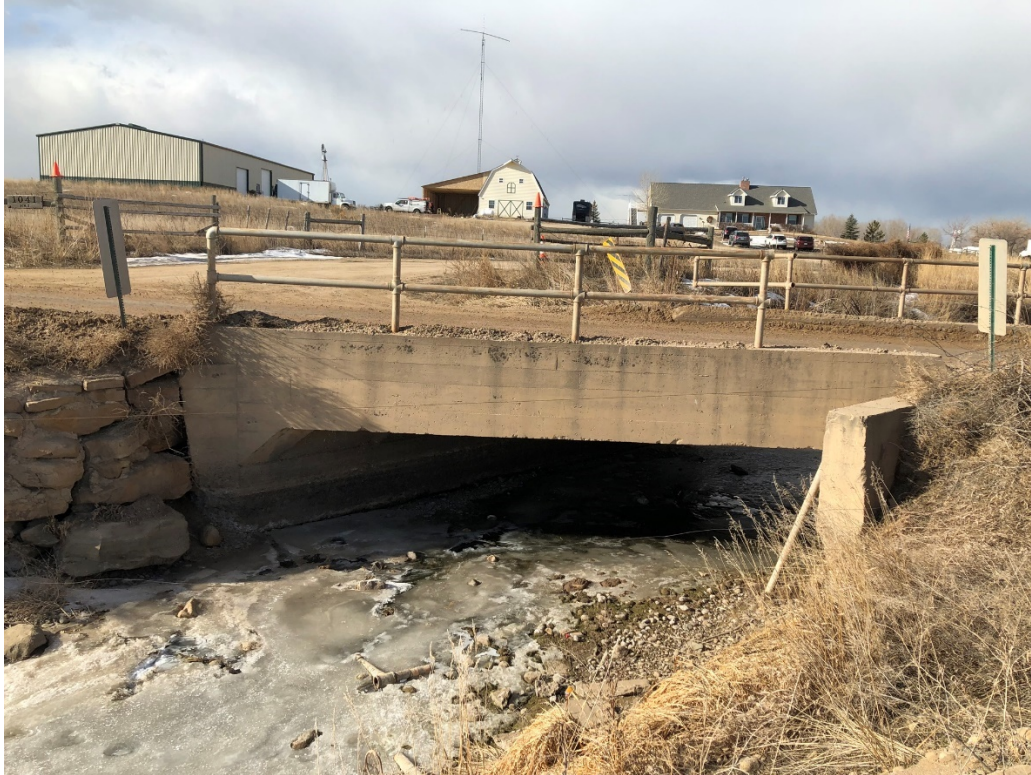
Figure 3 - Existing Structure at Hillsboro Ditch
